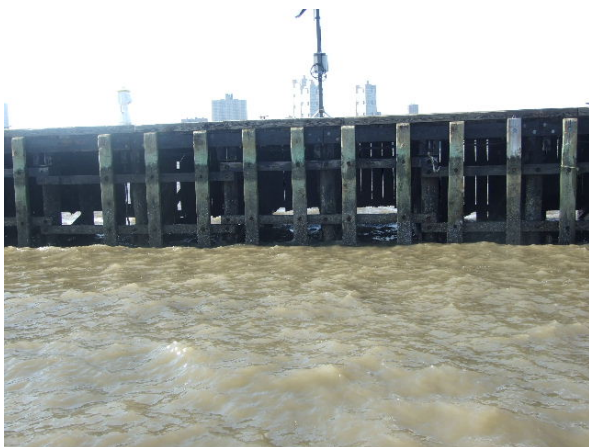
Wave wall from inside the Basin
