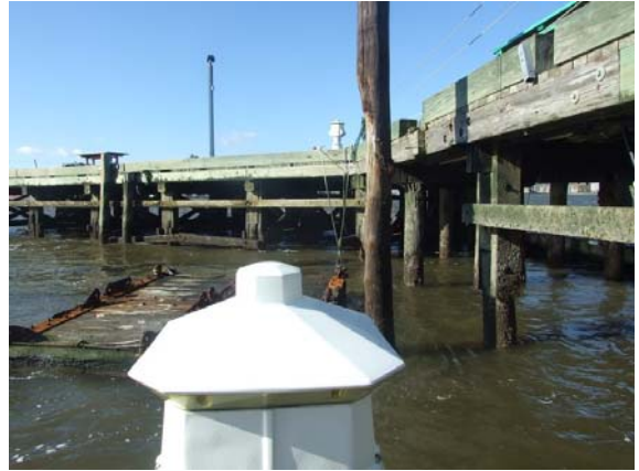
The pictures above show the daylight visible through the gaps of the A Dock head.
